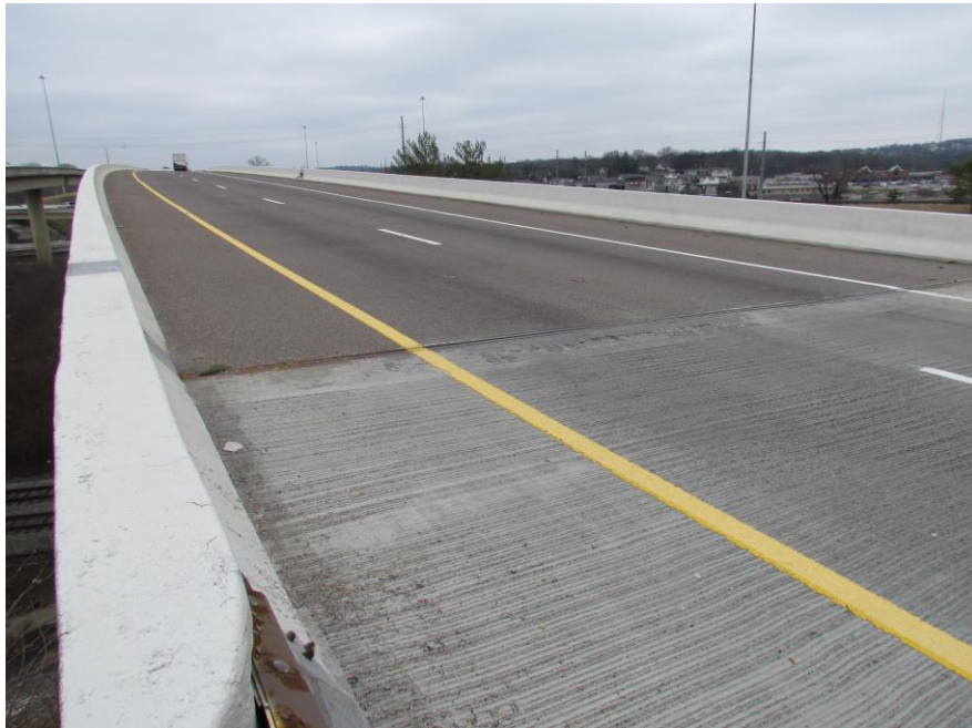
VIEW ACROSS TOP OF WEARING SURFACE
