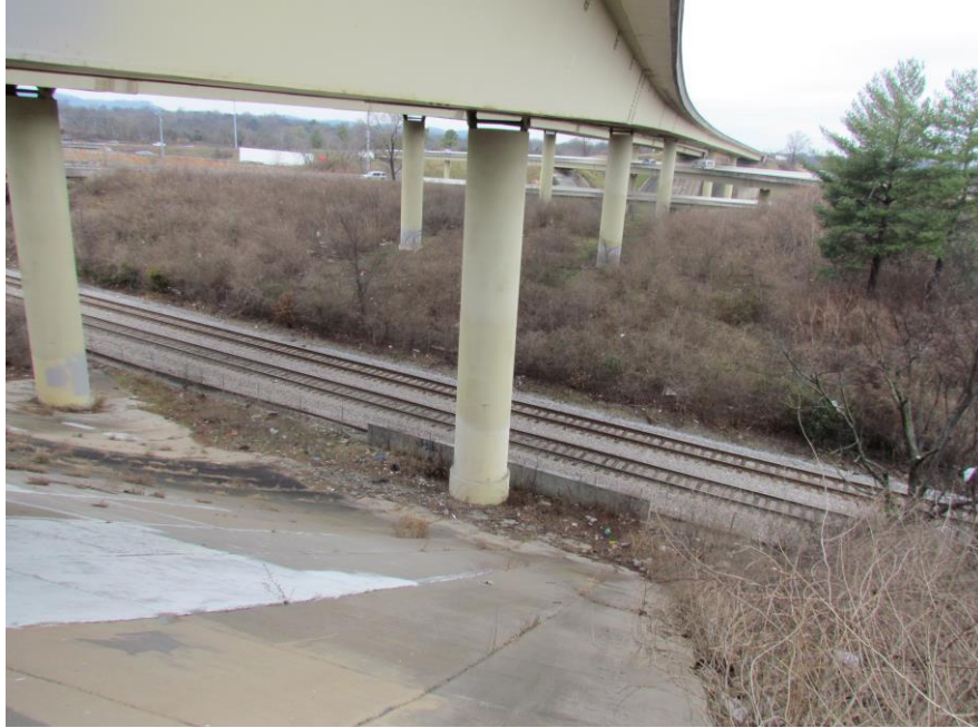
BENT #6 - BACK VIEW
