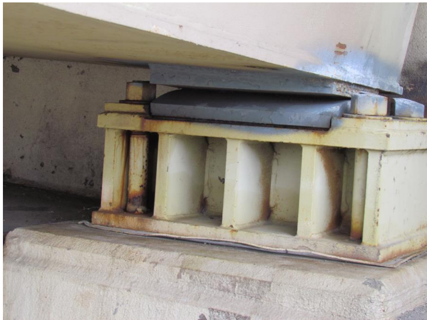
BEARING DEVICE "A" ABUT. #1 W/ REPAIR
