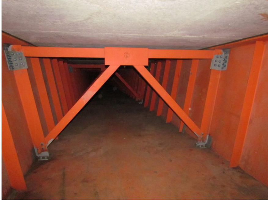
TUB "B" SP. #1 DIAPHRAGM #1 W/ REPAIRS TYP
