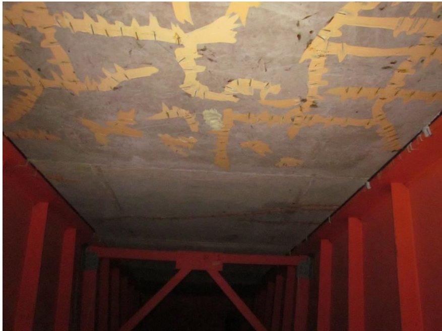
TUB "B" DECK PANELS SP. #3 W/ REPAIRS
