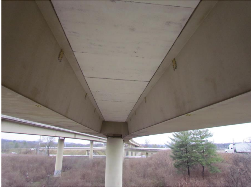
UNDERSIDE VIEW SPAN #6
